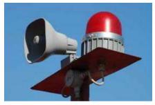
Alarms, sirens, lights, gauges and sensors continue to be important and widely applied technologies for warning and alerting at many facilities and hazard environments. Sites that use hazardous materials often install multiple systems that immediately warn onsite personnel and can further extend warning to neighbors and nearby facilities. River gauges on streams and motion sensors at dam sites are linked
