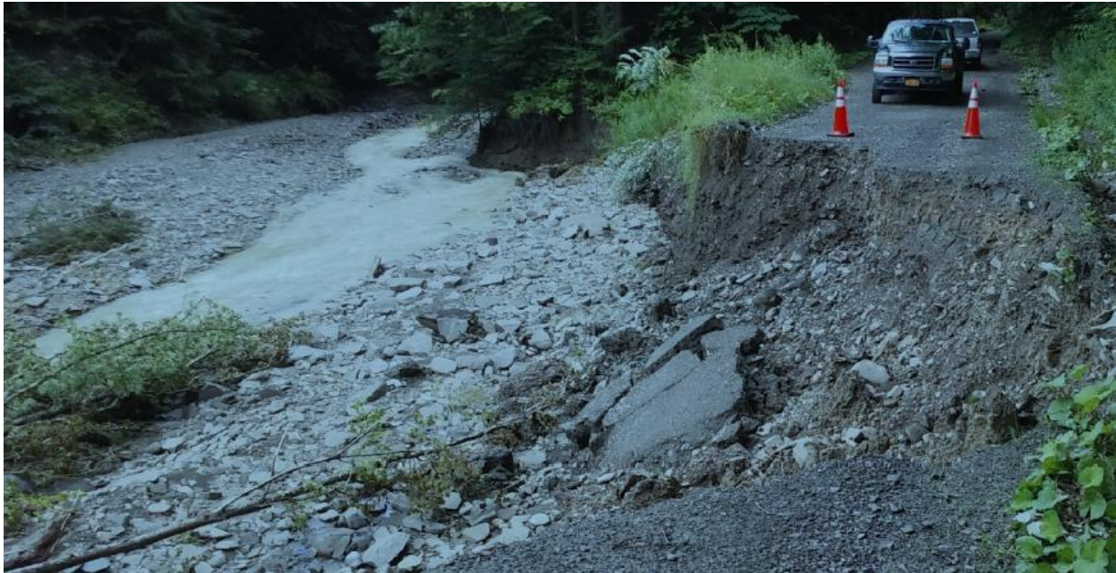
Figure 5.4.1-1. Flash Flood damages at Lower Briggs Hollow Road after July 2017 flash flood event.
