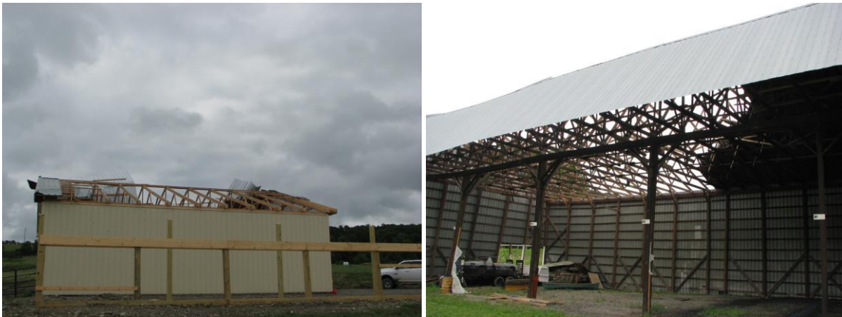
Figure 5.4.2-3. Microburst/Straight Line Wind Damage near Barton, July 2012
